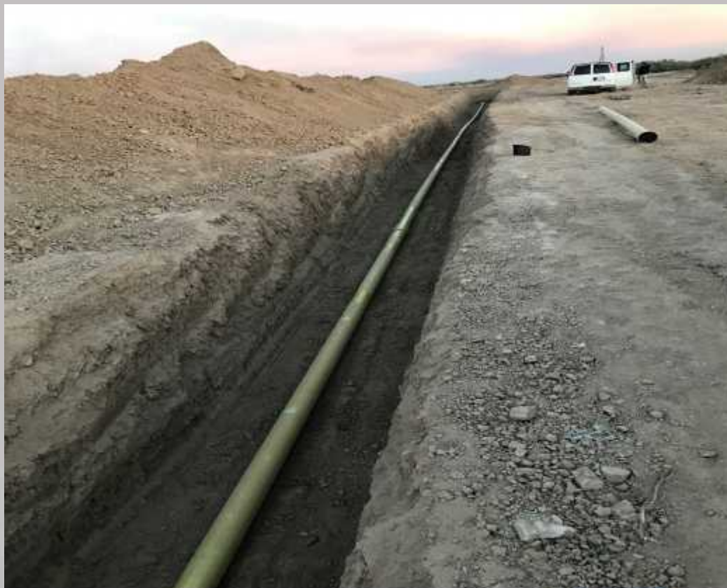
GRE PIPELINE EXCAVATION TRENCH
