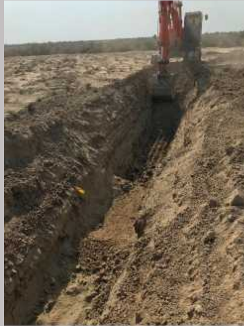
GRE PIPELINE EXCAVATION TRENCH
