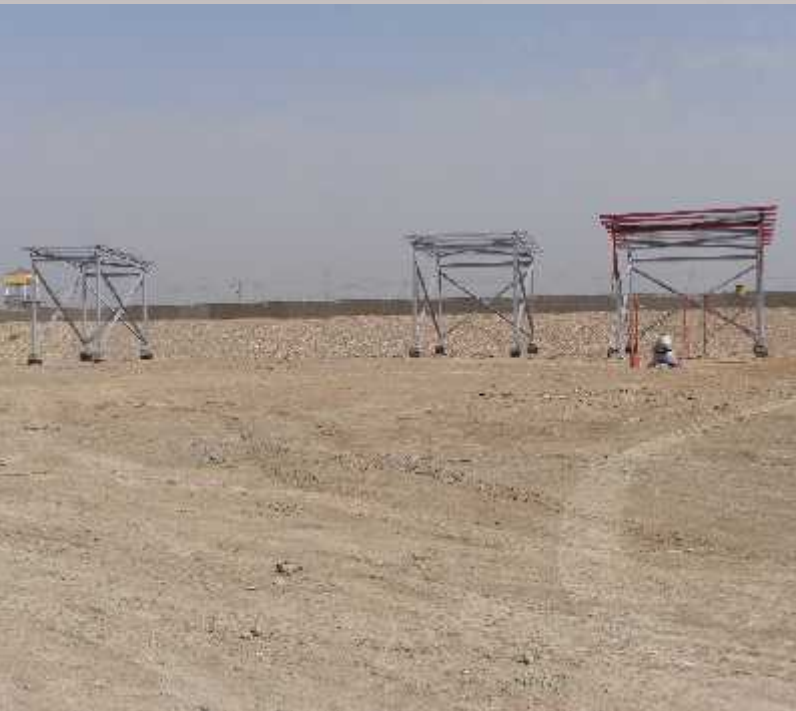
GENERATOR & TRANSFORMER SUNSHED
