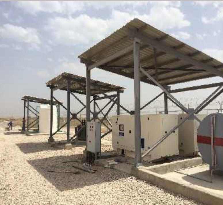
GENERATOR & TRANSFORMER SUNSHED
